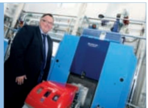
With variable outputs from 78kW to 1200kW Buderus cast iron boilers make an ideal replacement where a fully condensing system cannot be accommodated in practical terms. Boilers are supplied in unassembled sections to assist transportation and installation in otherwise difficult whilst confined spaces and front access via a hinged burner door makes servicing and maintenance straightforward.
